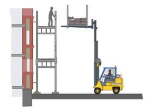
The materials are handled using a fork lift truck or similar. You can also use barrows at the site where the scaffolding is to be erected.
